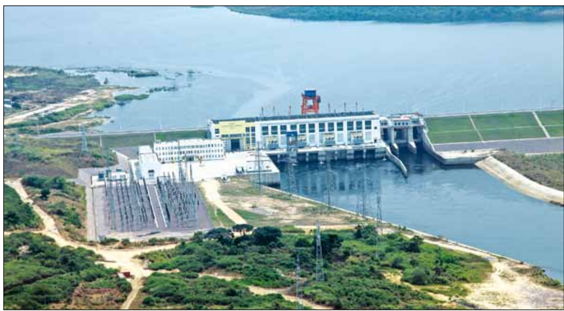
Imboulou Hydroelectric Power Plant.
