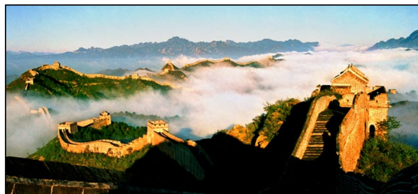
A restored section of the Jinshanling Great Wall in Hebei province.
